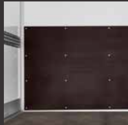
Front wall reinforcement
